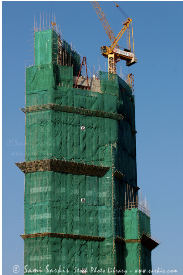
Scaffolding in construction
